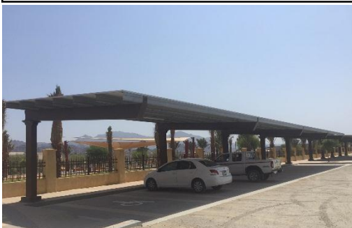
Dubai Municipality, Hatta, 120 kWp
