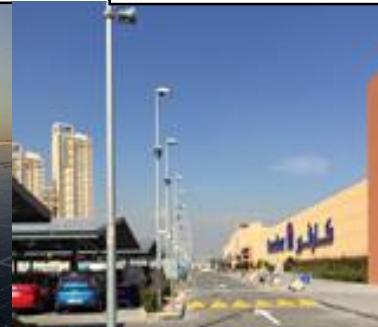
City Center Me'aisem, Tecom, 474 kWp
